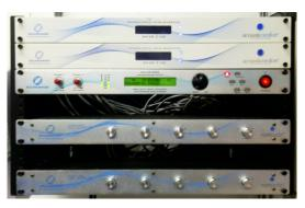
Soundmask system components neatly secured on a rack unit
