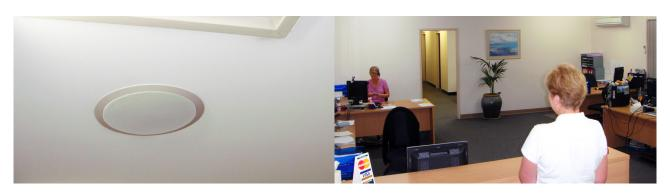
Soundmask's "cut in" transducer SM-TC-1265
