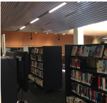
Pressed aluminium ceiling required expert
