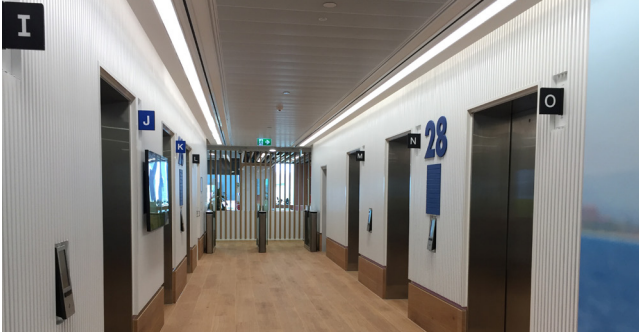
Foyer had pressed aluminum ceiling
