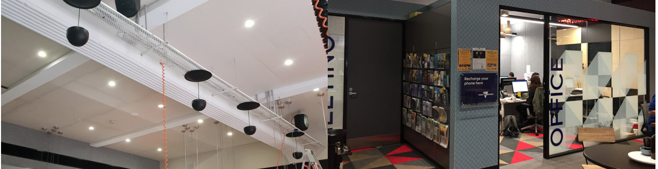
Transducers and acoustic discs suspended from the ceiling
